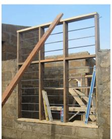
The process began with designing the housing. There it progressed from digging and laying the foundations to building up the floor, walls and windows. When the vertical planes were complete it was time to add the roof and shading devices onto the house.
