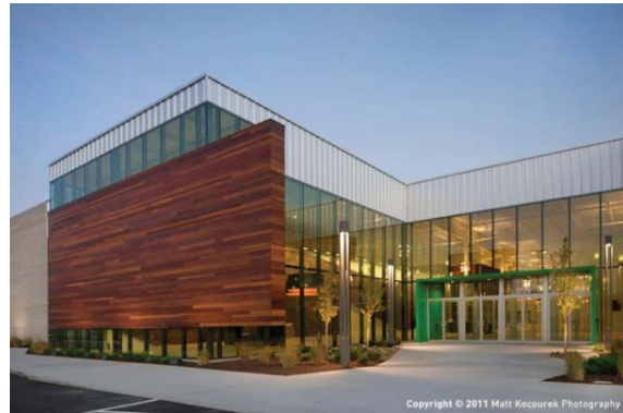
Figure 4: Exterior view of the church.
