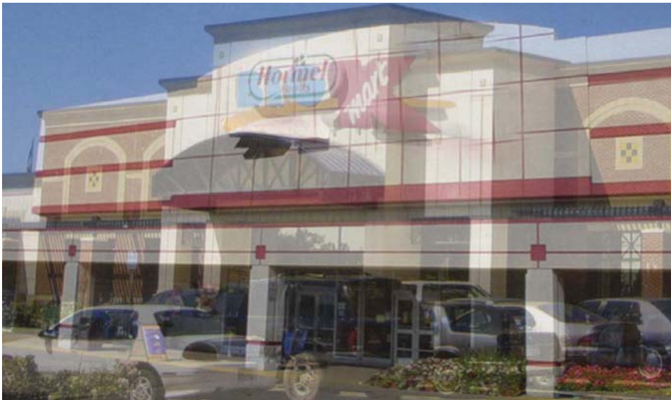
Figure C. Former K-Mart building is now Hormel Corporate's entrance
