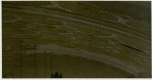
Figure 9 - Photo of Stony Island Arts Bank showing detail of patching missing plaster coffered ceiling with smooth layer set back
