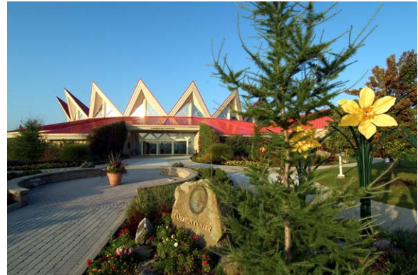
Figure 5. Entrance view of the Tamarack.
