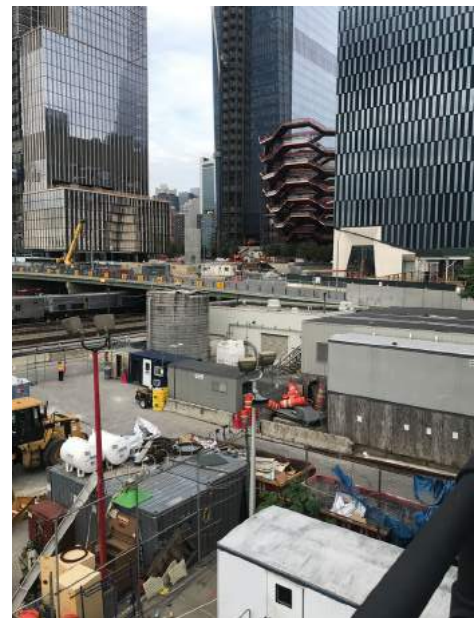
VIEW TOWARDS VESSEL
