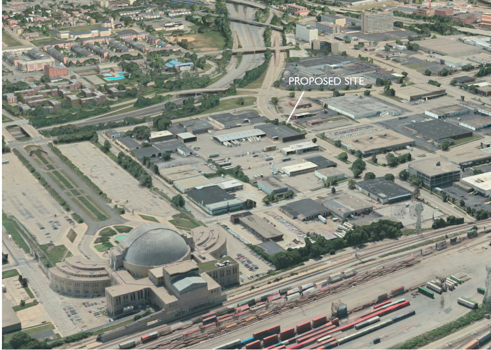
Initial Site Aerials
