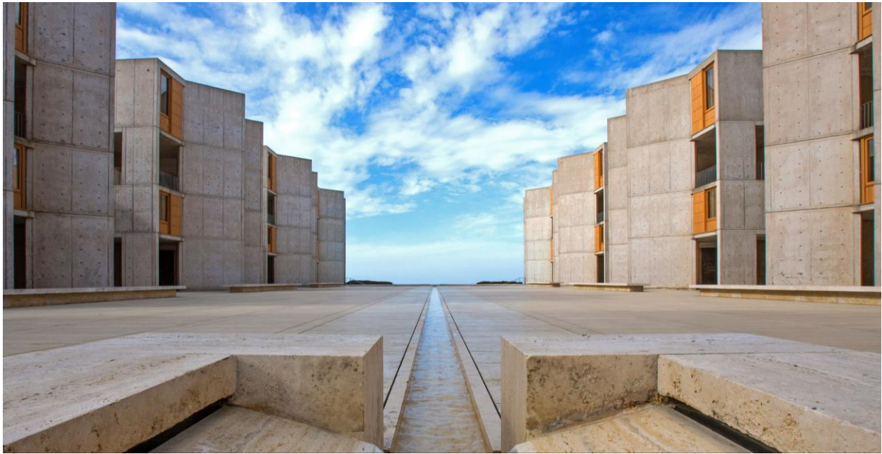
Fig 05: The buildings of the Salk Institute Established in 1960 by Jonas Salk, California, US
